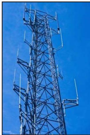
Figure 9-5 Repeater Antenna
